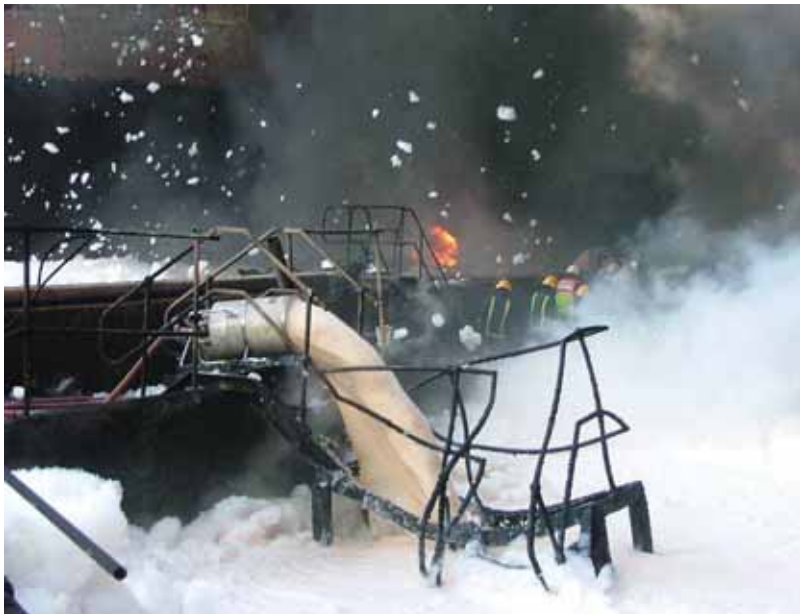
Angus foam pourers establish a foam blanket within the bund.
